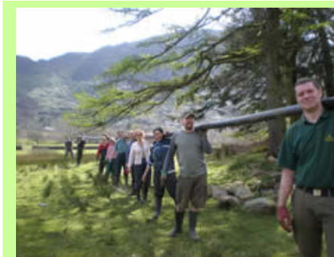
Working holiday installing micro-hydro pipe
